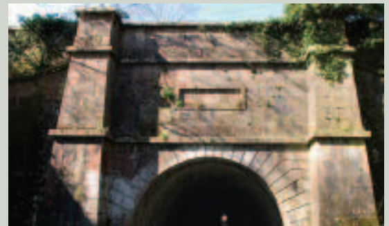
Grand: Hincaster Tunnel, East Portal
