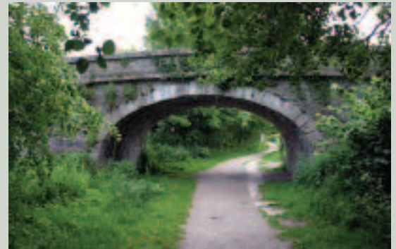
Canal footpath: Natland Mill Beck Lane
